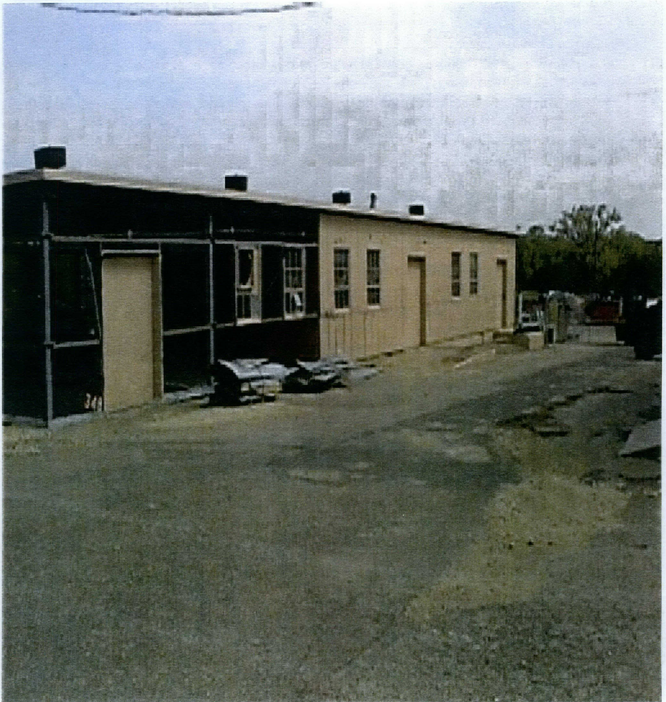
Figure 5 Digital Image of Pesticide Storage Facility
