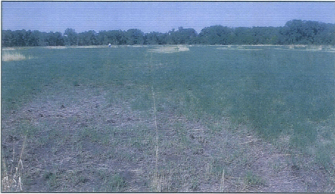
Photograph SFL2009-5 – View looking west of differential settlement in central portion of east half of landfill (11 May 09).
