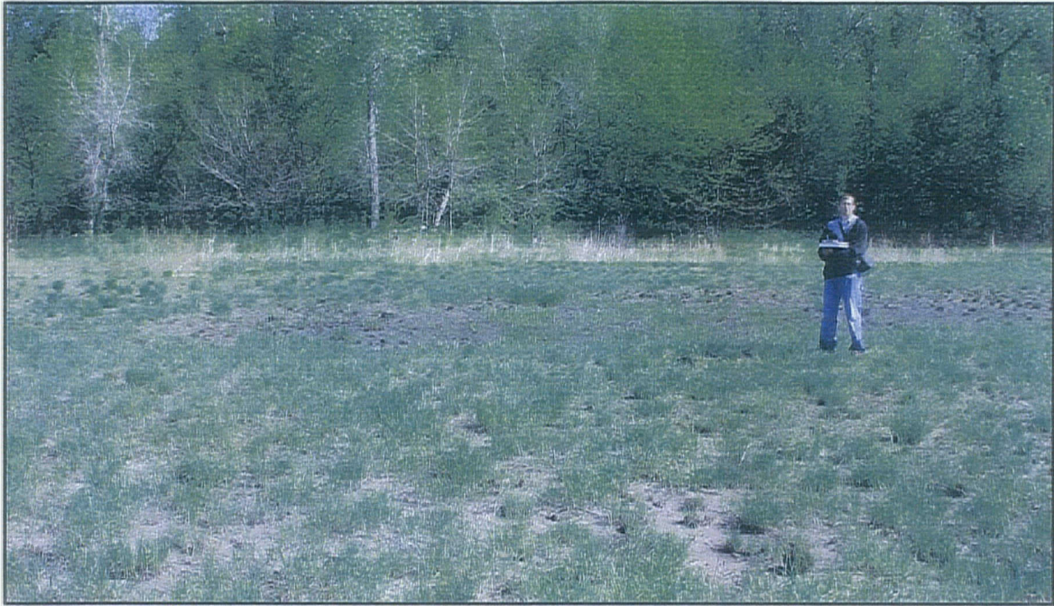
Photograph SFL2009-7 – Differential settlement/ponding at east central edge of landfill (11May 09).
