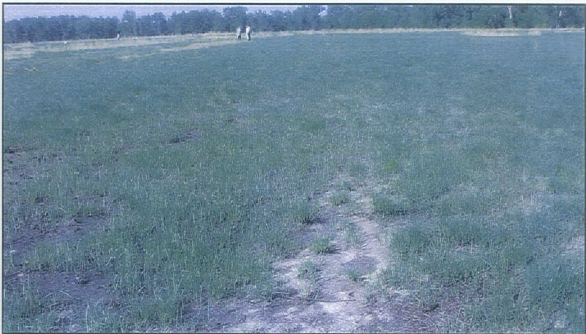
Photograph SFL2009-4 – View looking west of differential settlement/ponding in east central portion of landfill (11 May 09).
