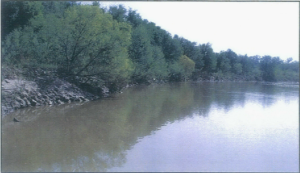
Photograph SFL2009-9 – Upstream reach of rock revetment (11May 09).
