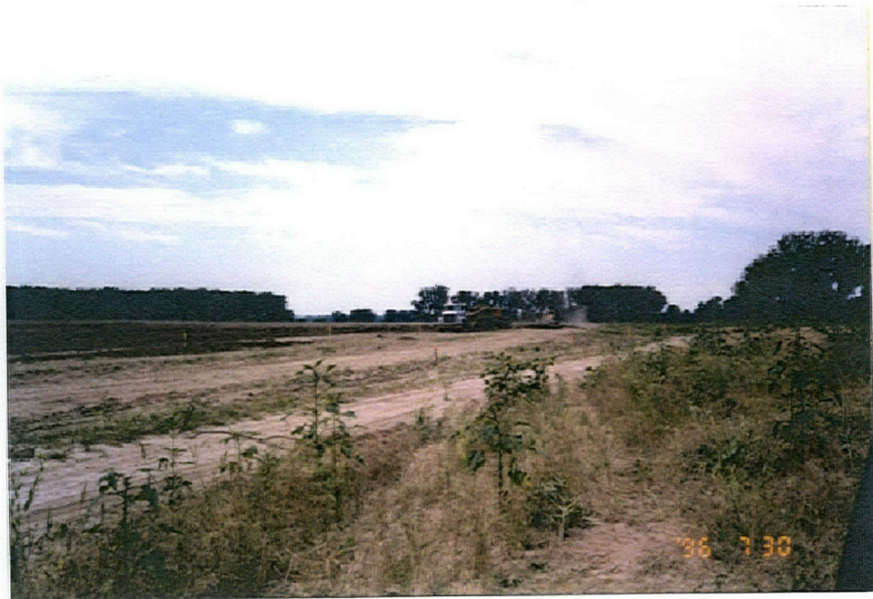
View of Native Soil Cover in southeast quadrant of landfill during placement of fill under Cover improvement Project (July 30, 1996).
