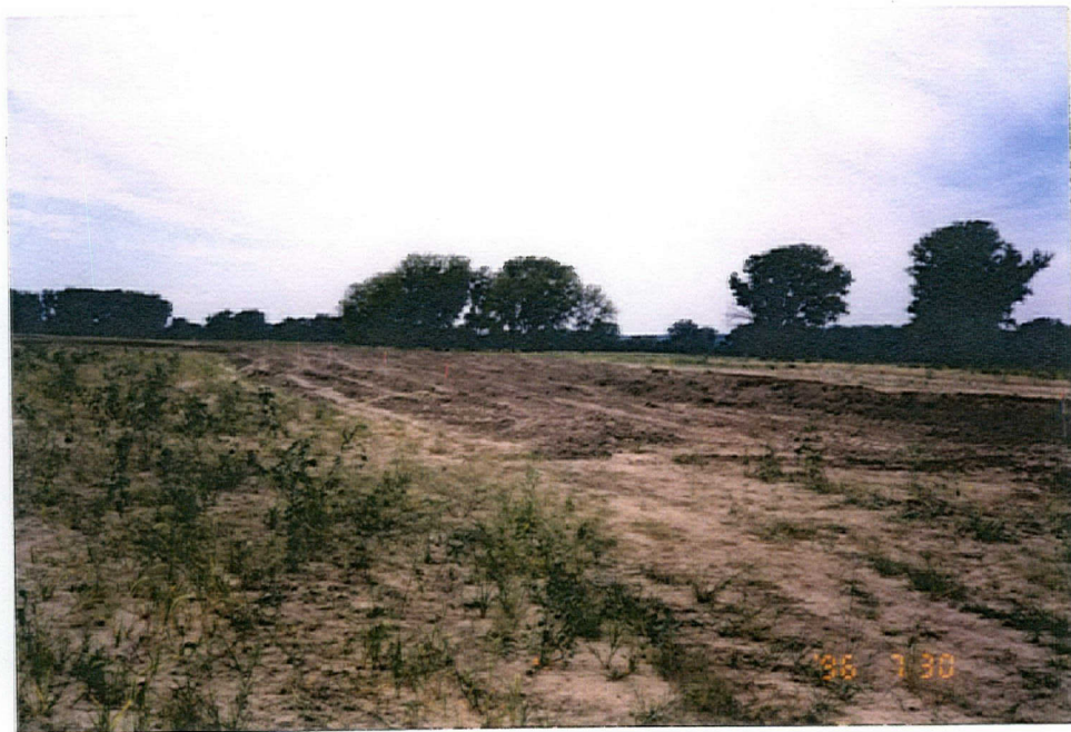
View of Native Soil Cover looking from southeast quadrant towards center of landfill. (July, 1996)
