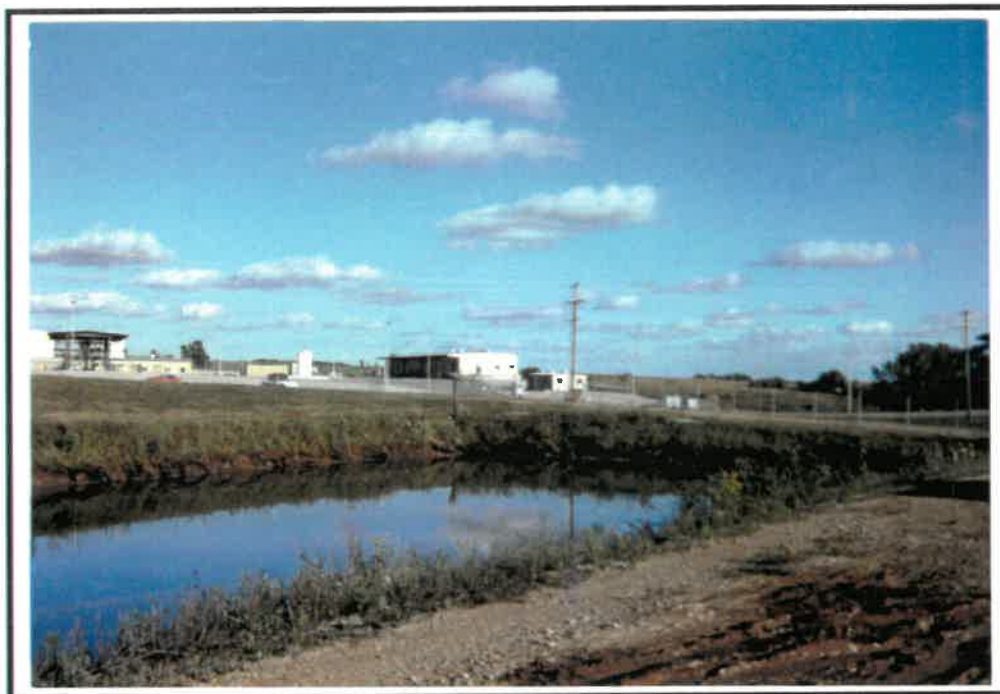
Photograph Number 12 East Pond -- From Sample Location D1, Looking Southeast Toward Fence Gate
