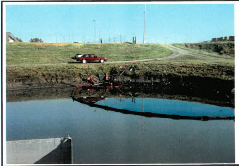
Photograph Number 7 West Pond -- Boom, Inlet Looking North
