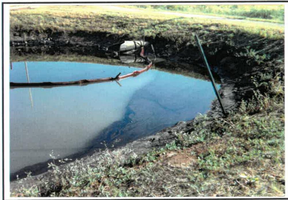
Photograph Number 8 West Pond -- Inlet/Booms Looking Northeast
