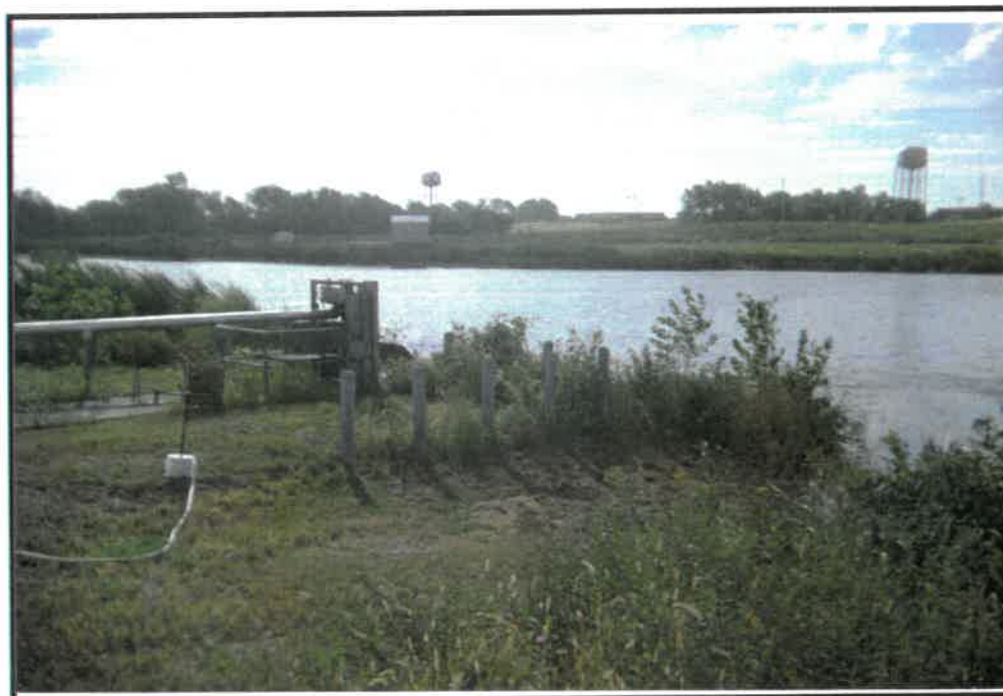
Photograph Number 14 Wash Rack Reservoir -- Outlet Sample Area Looking Southeast
