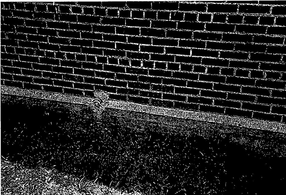
CAPPED VENT LINES - END OF PROJECT
