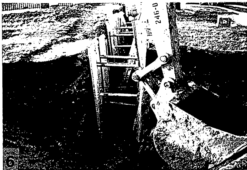
6 EXCAVATION AFTER THE MANHOLE OVERFLOWED - MIDDLE OF PROJECT
