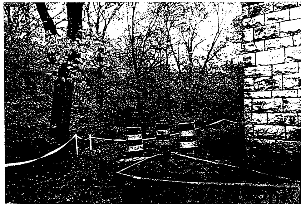
WATER DIVERSION FROM OVERFLOWING MANHOLE TO NEXT MANHOLE - MIDDLE OF PROJECT
