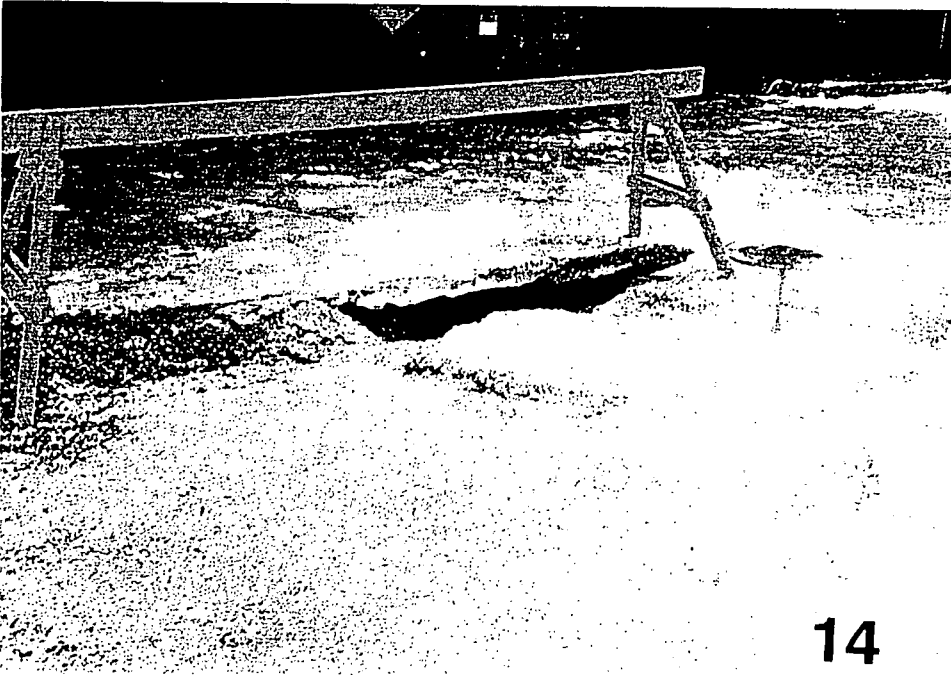
WASHOUT NEAR LOWER MANHOLE - NEAR END OF PROJECT
