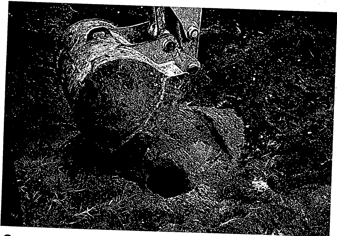
IN-PLACE ABANDONMENT OF LARGE UST - NEAR END OF PROJECT
