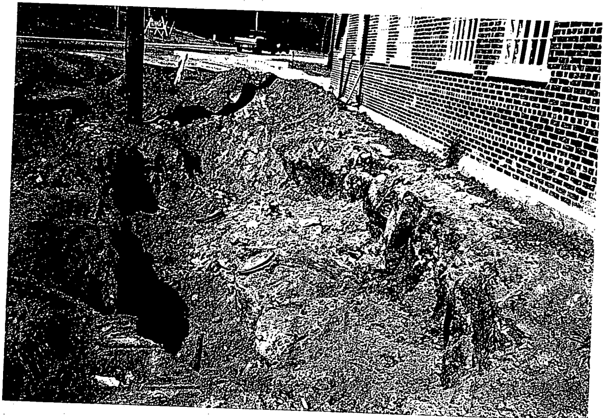
TOPS OF USTs AND PIPING - MIDDLE OF PROJECT
