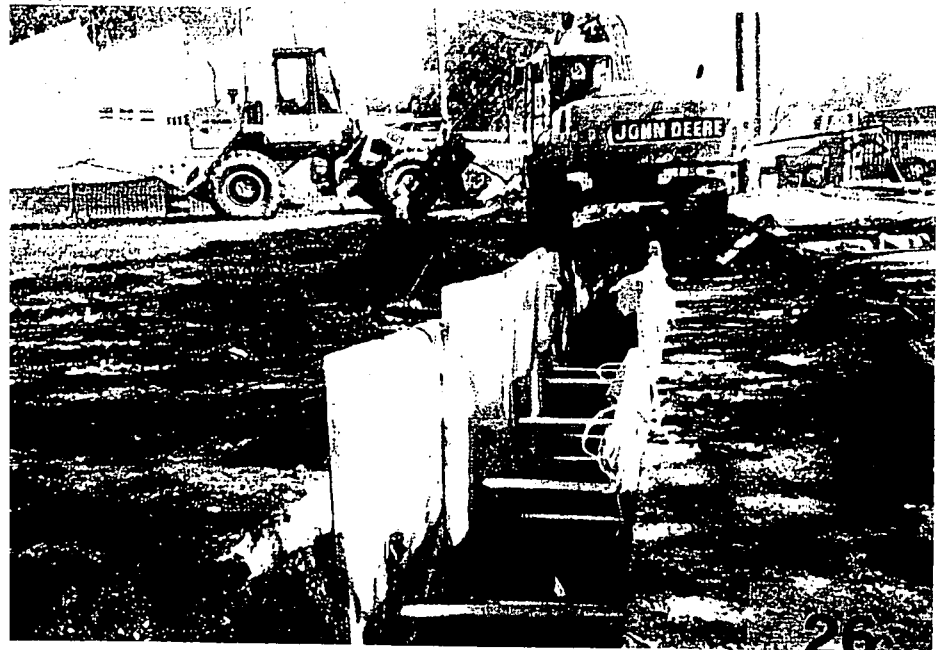
HYDRAULICALLY-JACKED ALUMINUM TRENCH SHORING - MIDDLE OF PROJECT
